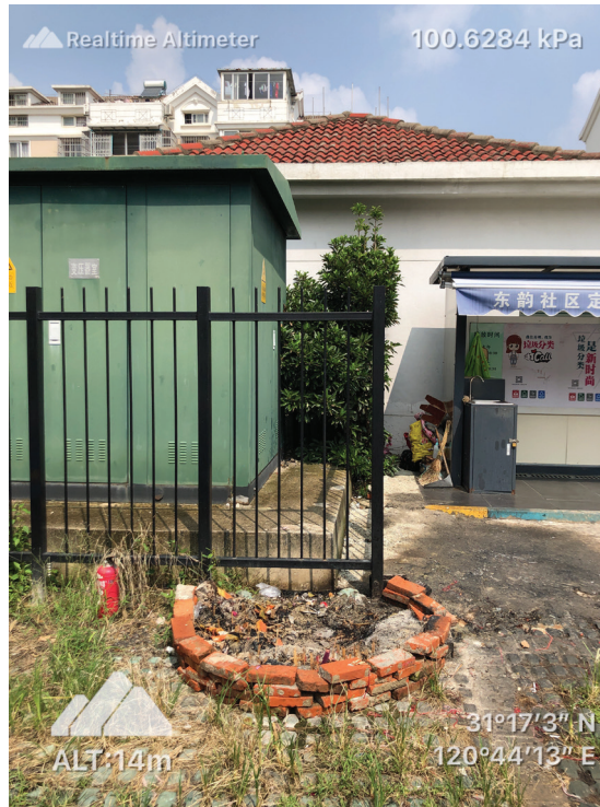
FIGS. 1A AND 1B Incense Burning Spot by a Parking Lot and Garbage Station, photos by Wenxuan Yang.
